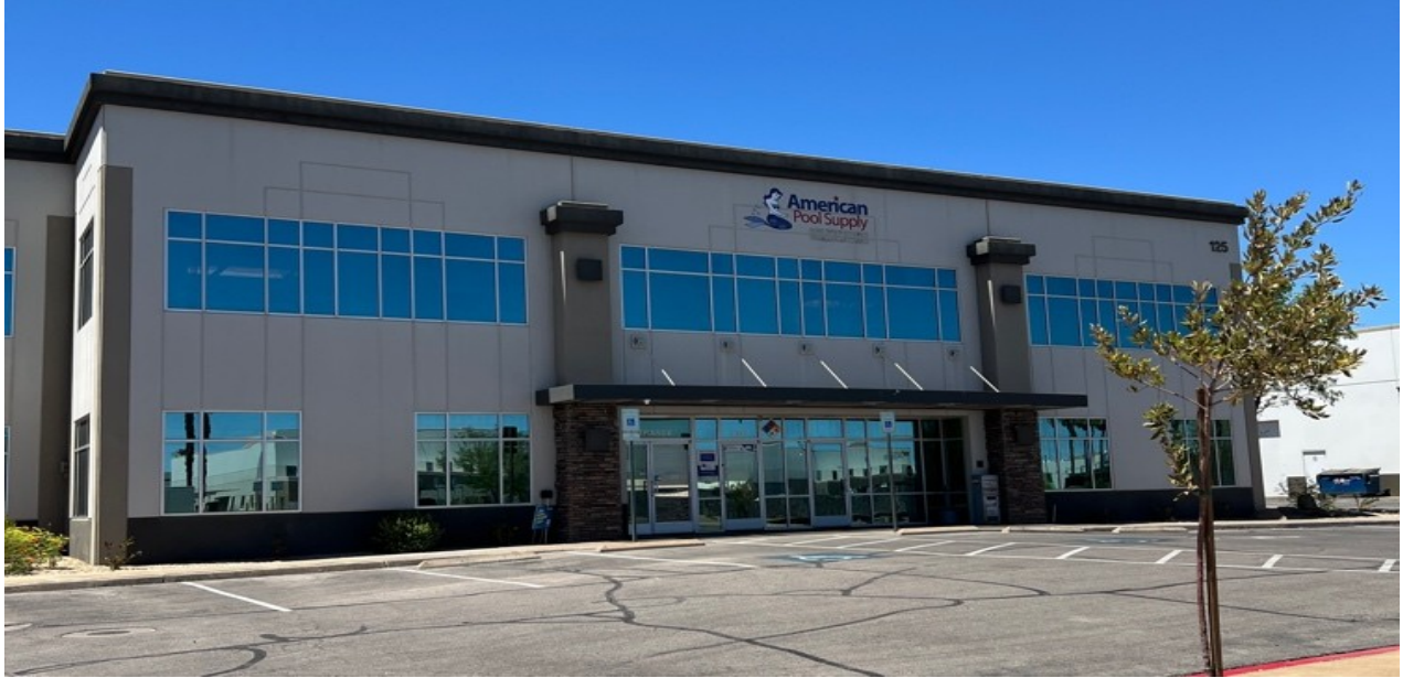
High Image 12,320 SF Freestanding Building
