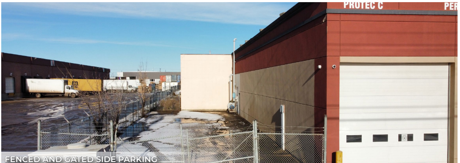
FRONT LOADING WITH 14' (H) X 12' (W) OVERHEAD GRADE
