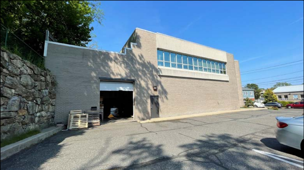
ONE DRIVE-IN DOOR ON LEFT
