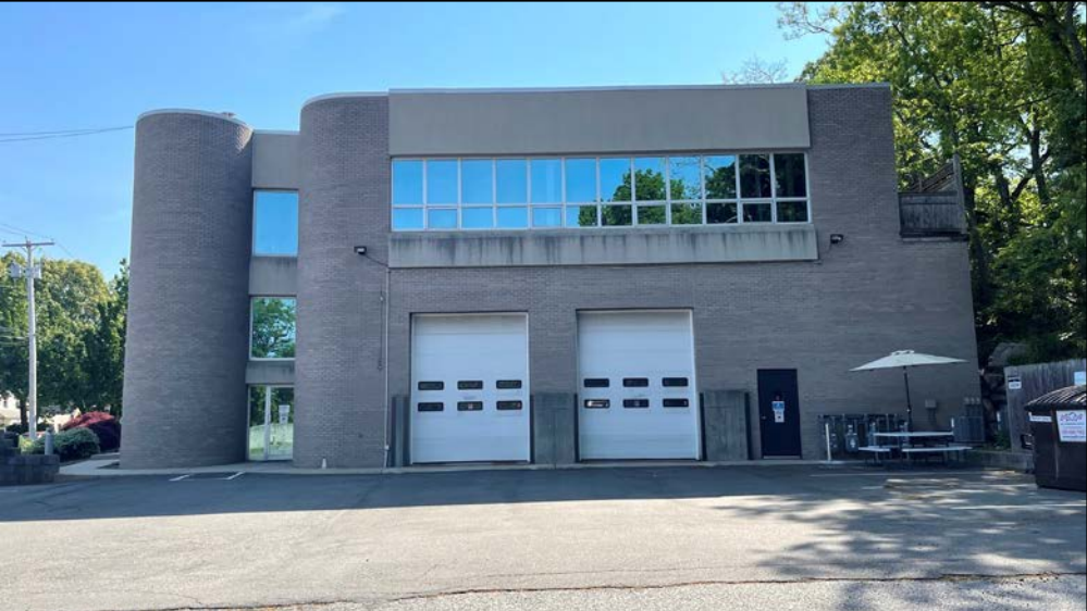
TWO DRIVE-IN DOORS ON RIGHT
