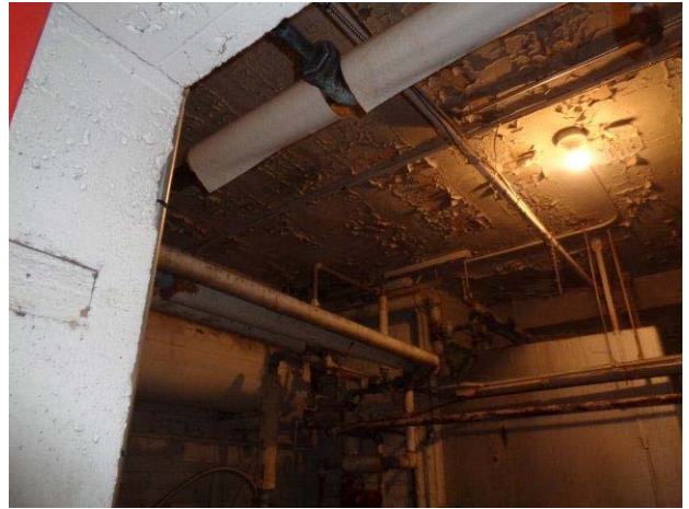
Garden Level Boiler Room Ceiling – Peeling Paint
