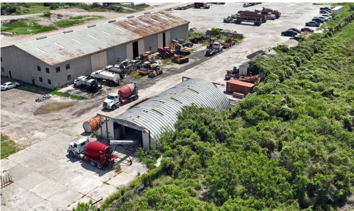
3. Quanset Building: 4,008 SF
