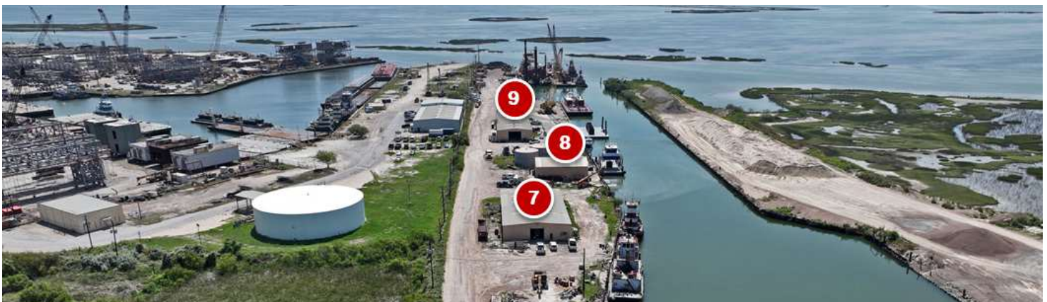
Building Structures No. 7 - No. 9
