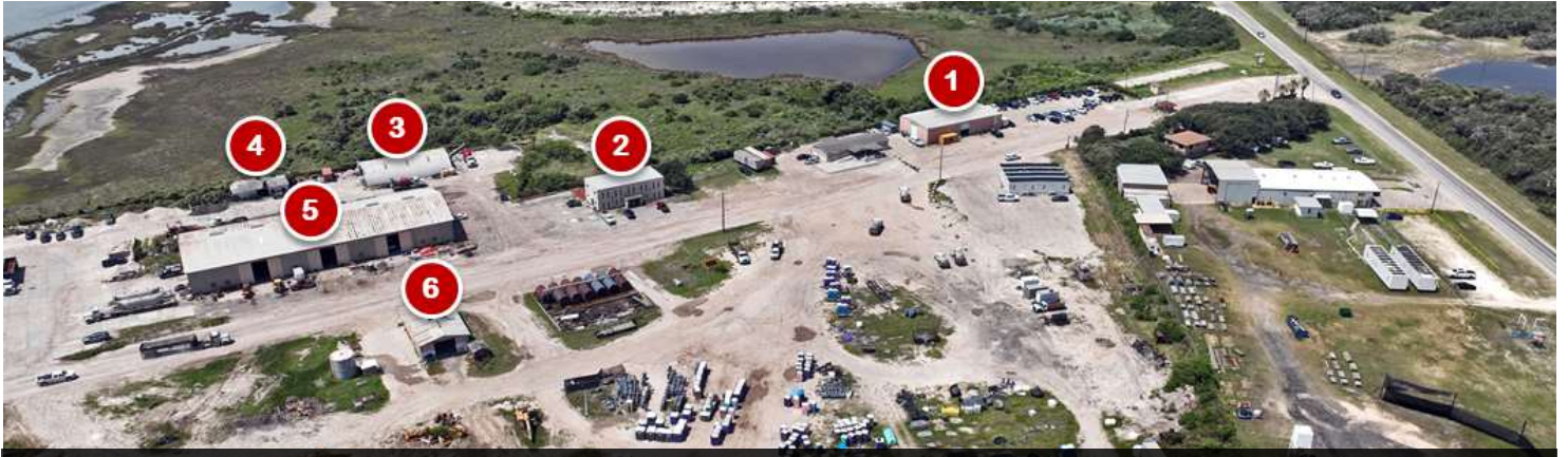
Building Structures No. 1 - No. 6
