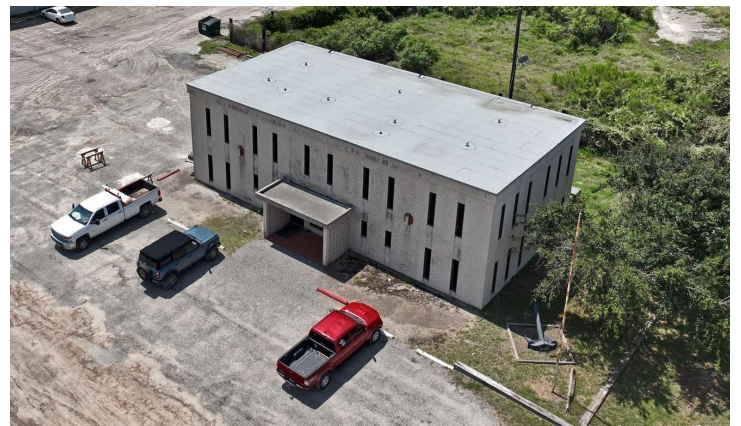
2. Garrett Construction Building: 4,888 SF
