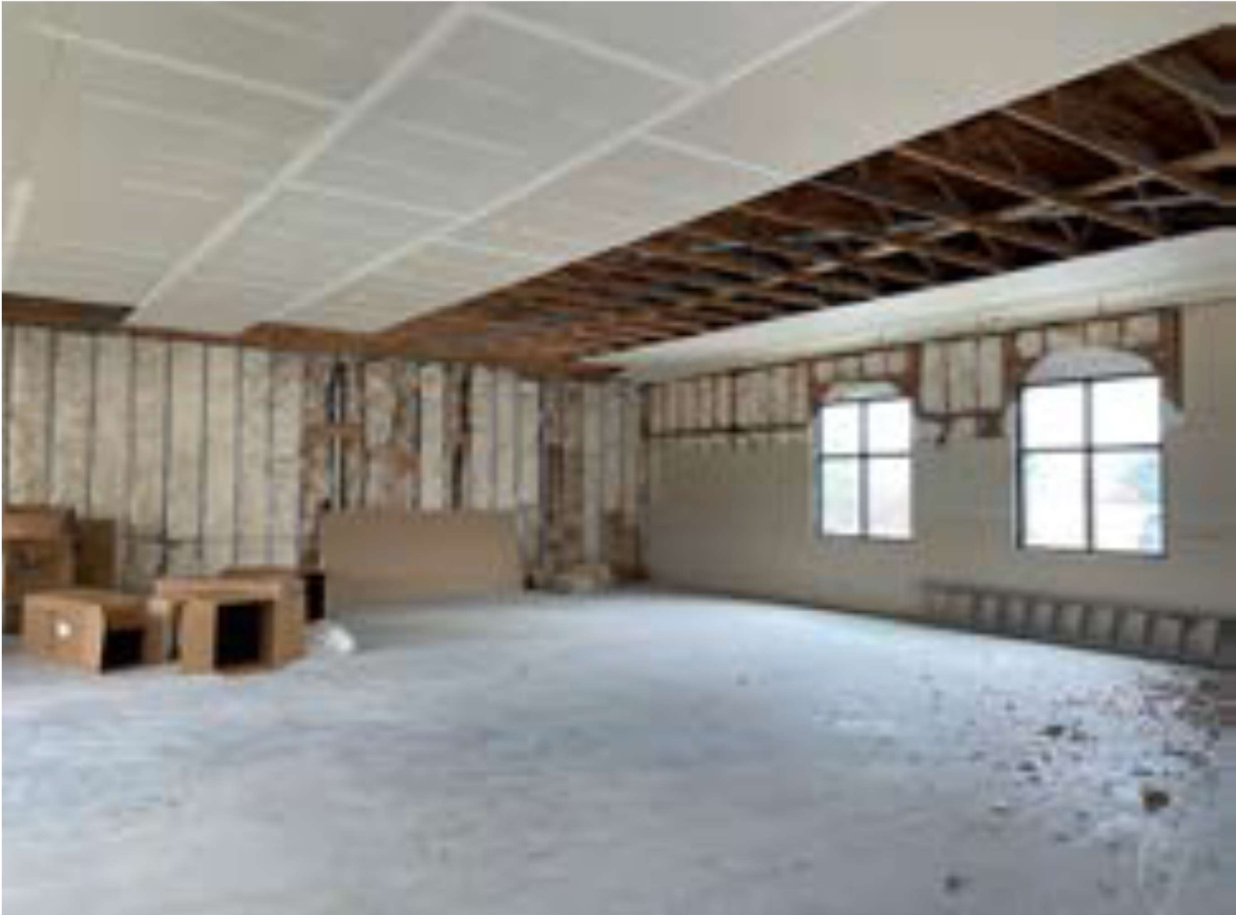
INTERIOR VIEW TO BACK WINDOWS / PARKING
