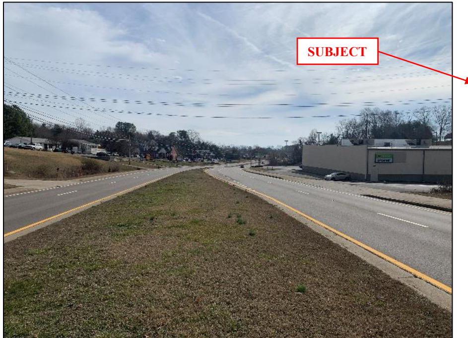
EASTERN VIEW MIDDLEBROOK PIKE (TN-169) AT MIDTOWN COMMONS WAY
