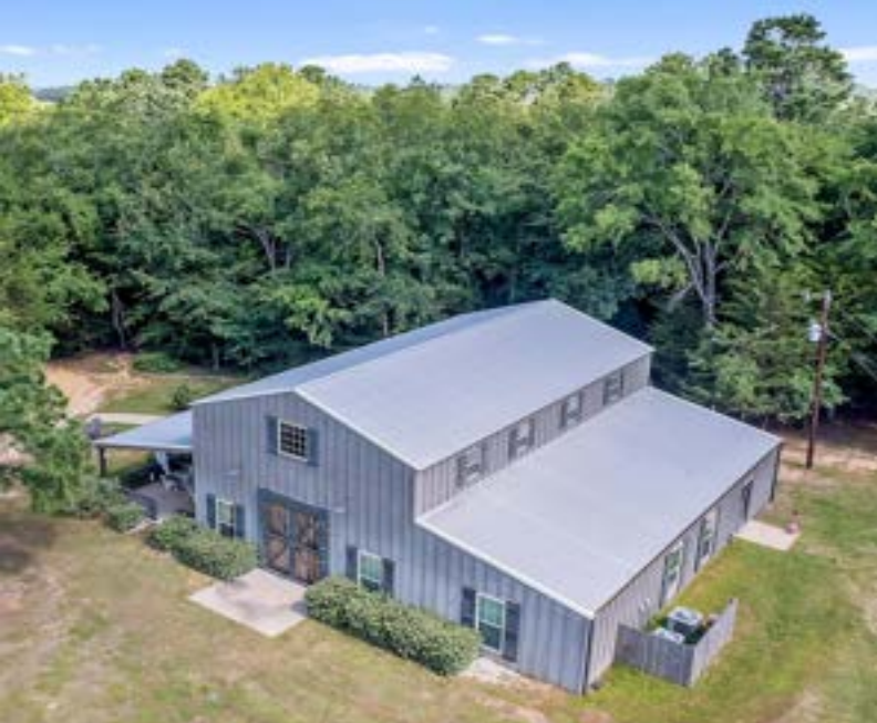
Dining Hall/Reception - 2 story with new flooring
