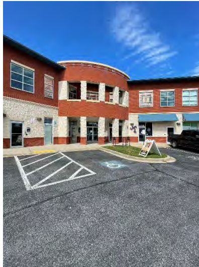
Entrance Door with Elevator
