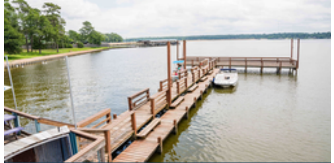
PIER + BOAT ACCESS
