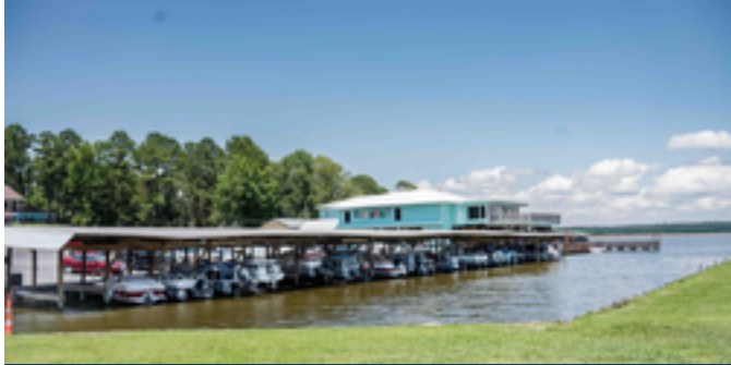
MARINA + COVERED SLIPS
