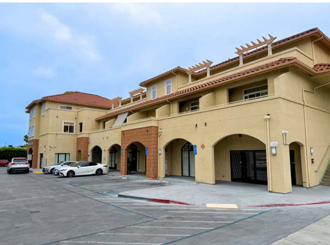
Exterior - Parking Lot
