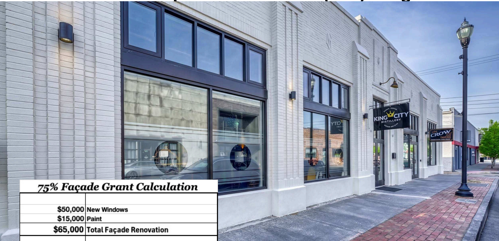
Facade Grant - Potential Renovation
