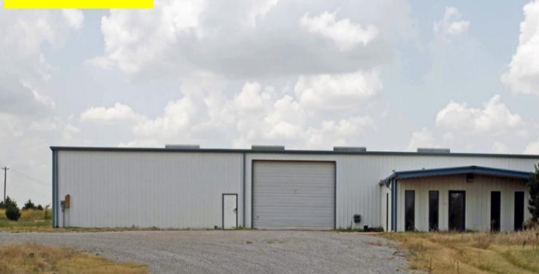
Front of warehouse
