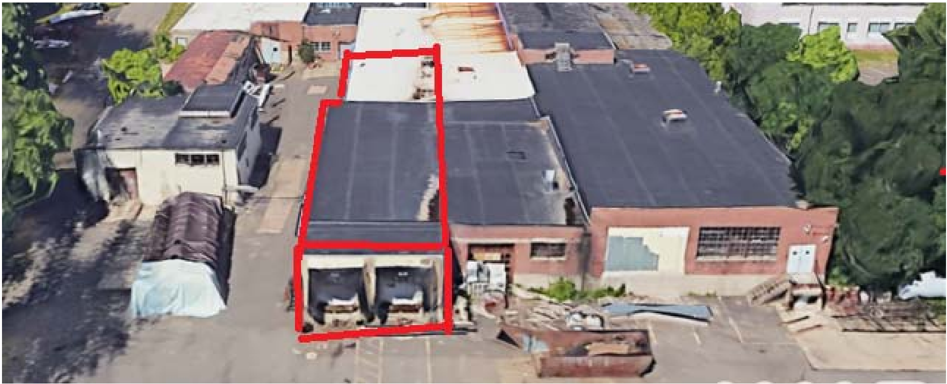
EXISTING BUILDING – FRONT – VIEW WEST FROM REAR – UNITS 3, 4, 5
