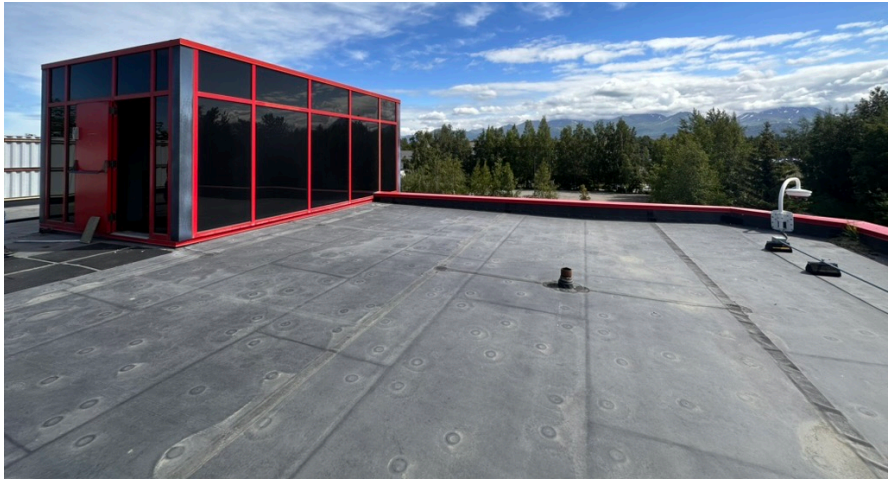
Roof looking East
