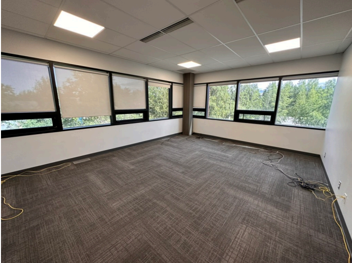
2nd Floor Renovated Offices
