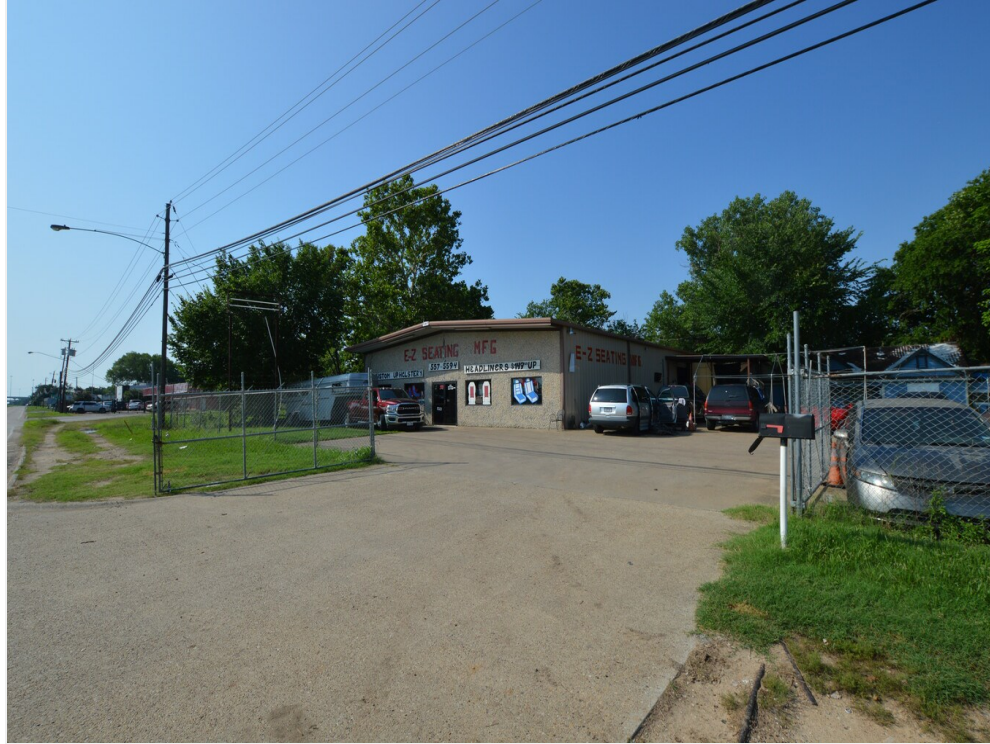
Front Elevation - Close up - 10426 (2)
