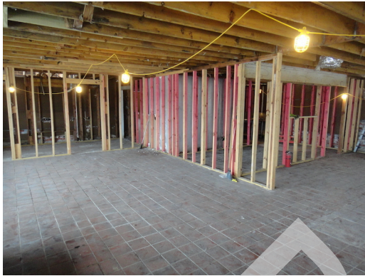
Interior overview bldg 1
