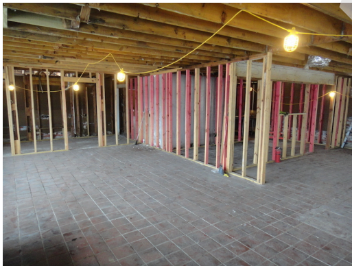
Interior overview bldg 1
