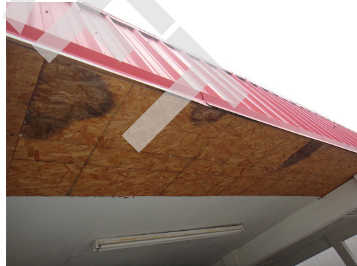
Damaged soffits
