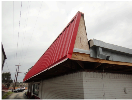
Roof parapet wall
