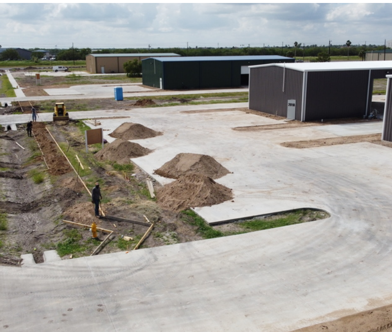
For Example Only - New Warehouses under Construction
