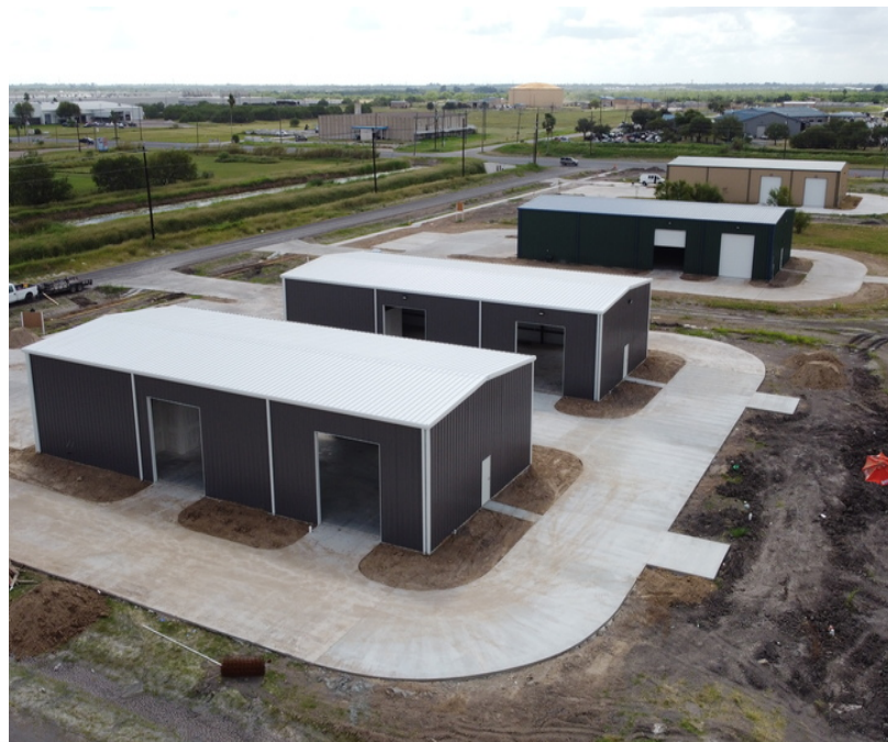
For Example only - New Warehouse under Construction
