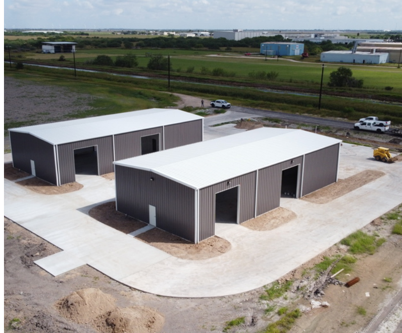
For Example Only - New Warehouses under Construction
