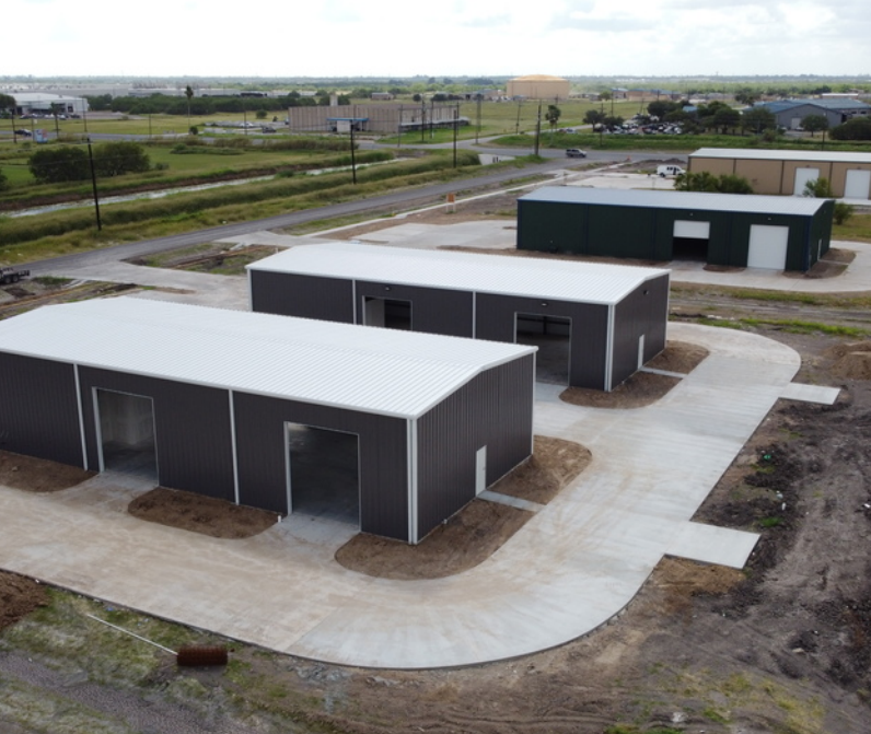
For Example Only - New Warehouses under Construction
