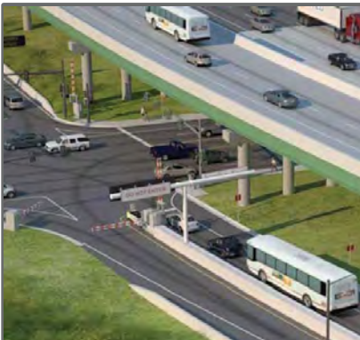
Northwest Corridor Express Lanes
