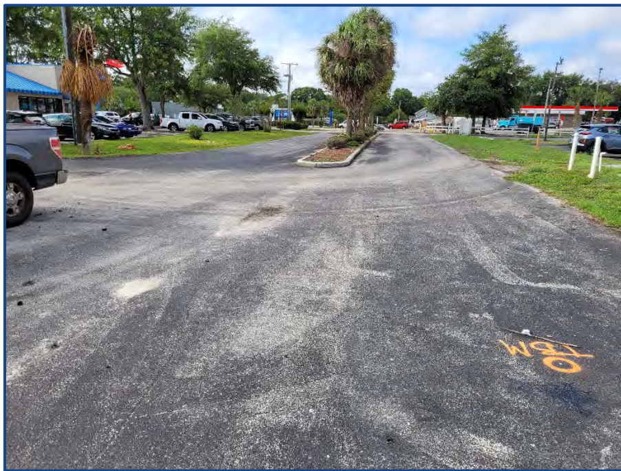
Photograph No. 2: Looking south at the entrance to the subject property.
