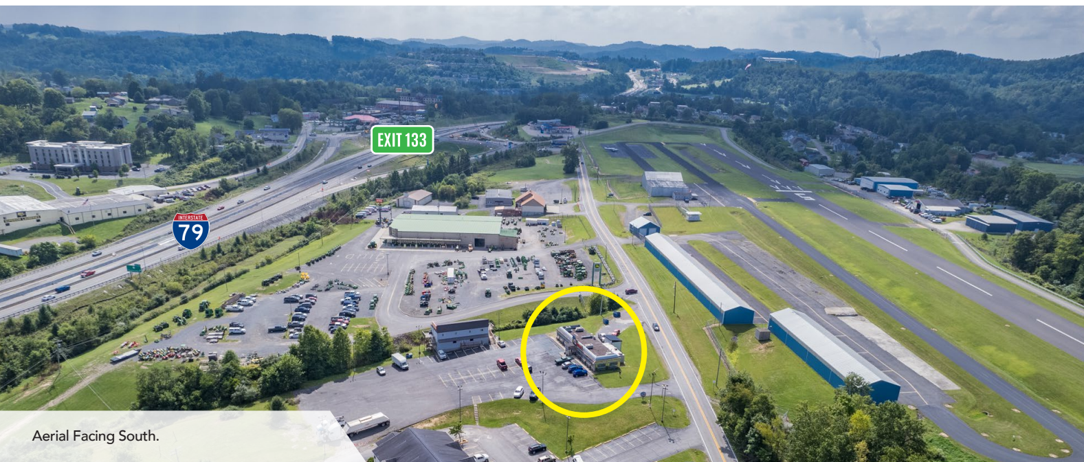
Aerial Facing North.
