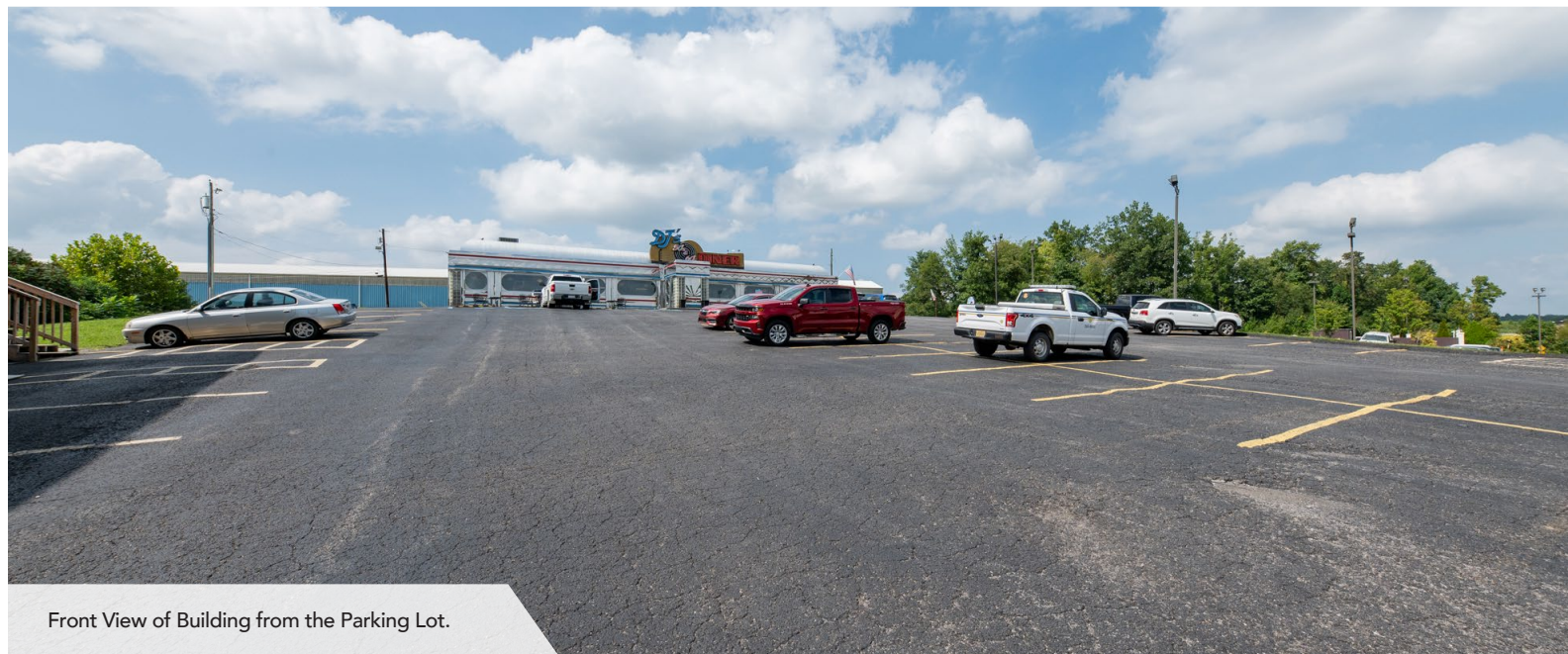
Large Parking Lot.
