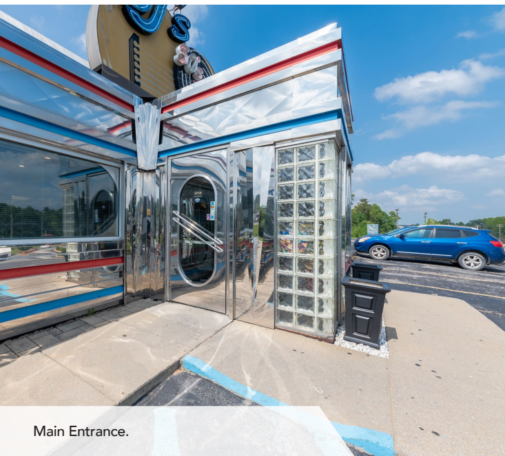
Front of Building.
