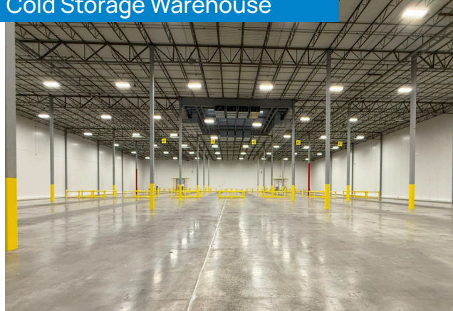
Cold Storage Warehouse
