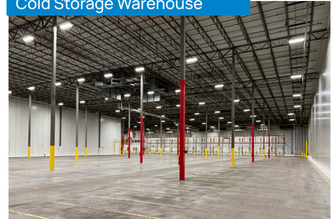
Cold Storage Warehouse
