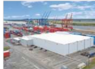
PORT OF WILMINGTON COLD STORAGE
