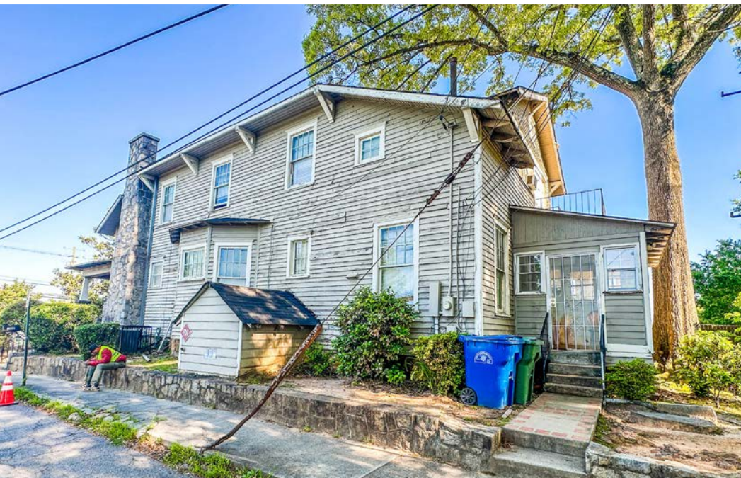
EXTERIOR PHOTOS (MAIN STRUCTURE)
