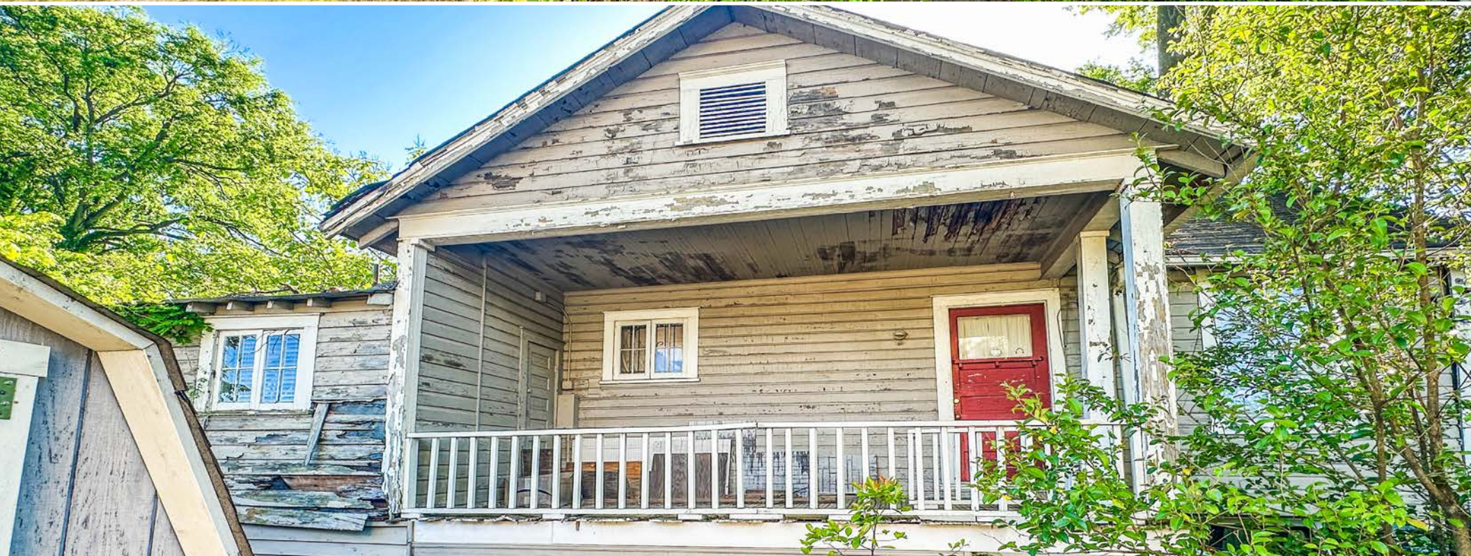
EXTERIOR PHOTOS (REAR STRUCTURE)
