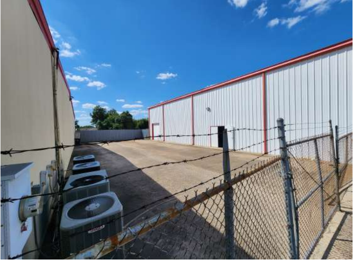
Secure storage between buildings
