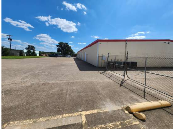
Large concrete parking area is in great condition
