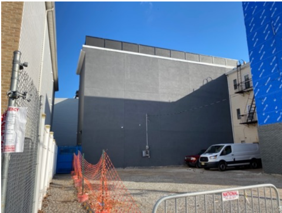
Side View from Leonard Street facing northeast
