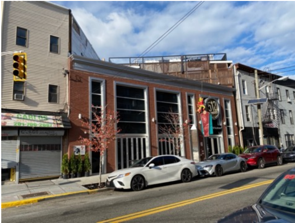
Front View from Paterson Plank Road facing west
