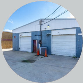
Two Rear Drive-In Doors
