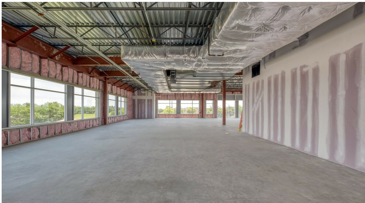
Spaces in Shell Condition Ready for Build-Out
