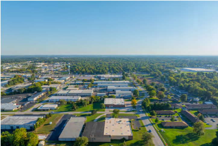
North Side Looking South
