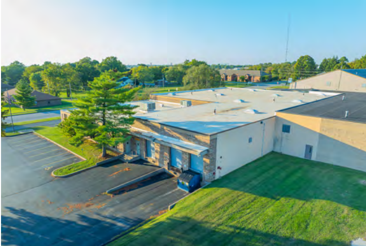
Southeast Looking Northwest
