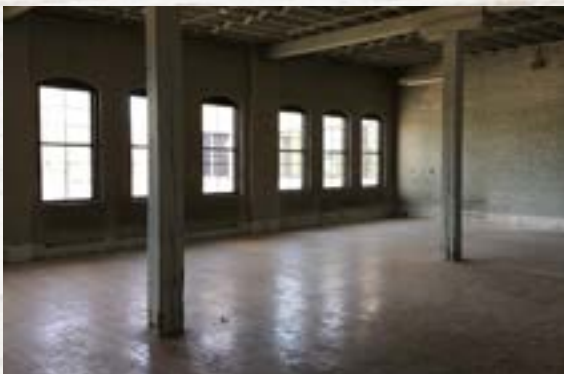
3rd Floor - Unfinished Space
