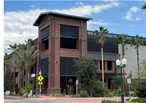
NEW 385 SPACE PARKING STRUCTURE WITH CHARGING STATIONS
