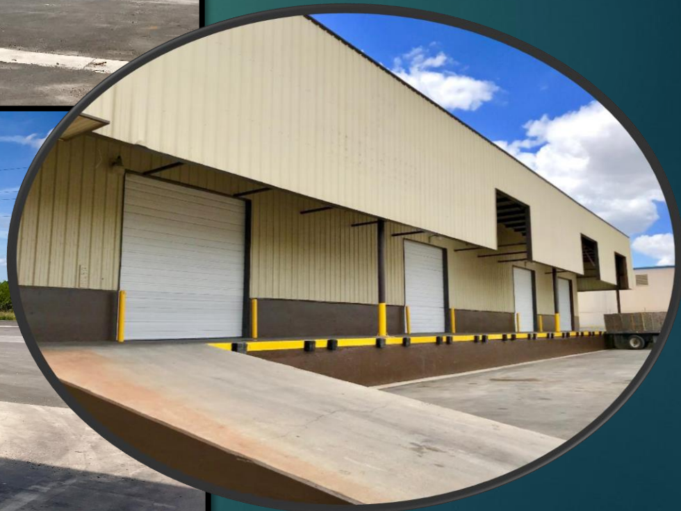
Front Covered dock
