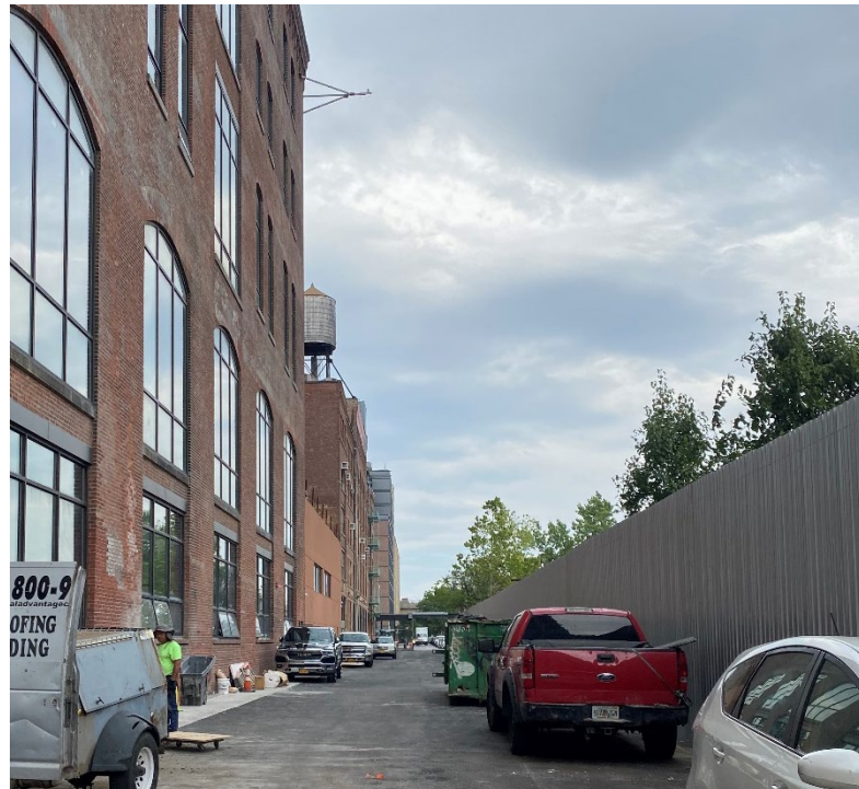
Potential loading area, rear of building
