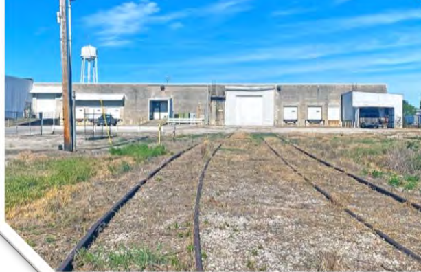
Rail Service to Section B
