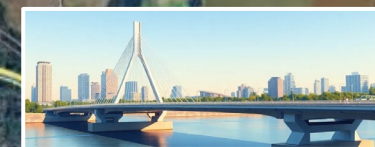
NEW I-55 BRIDGE
