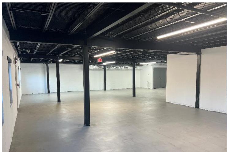
Example Finished Space (Suite 101)
