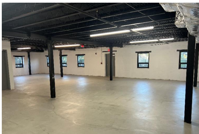
Example Finished Space (Suite 101)
