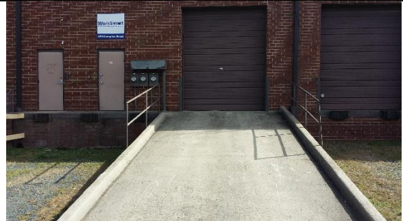
Concrete roll in dock ramp
