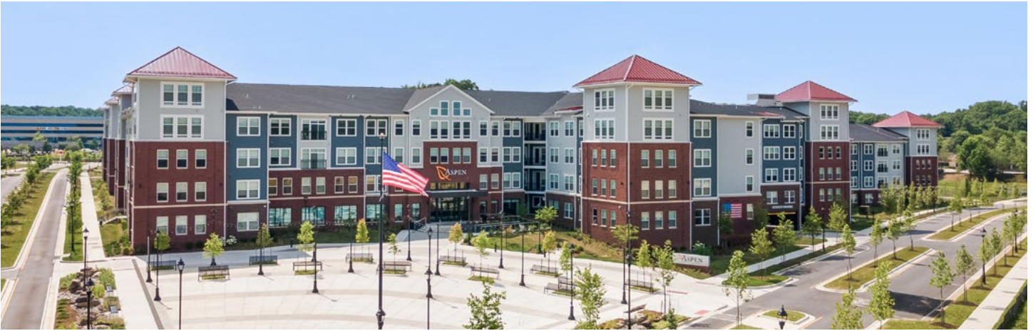
Aspen at Melford Town Center: Now Open
