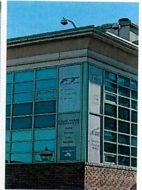
Exterior signage for tenants
