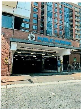
Parking garage behind the bldg.
