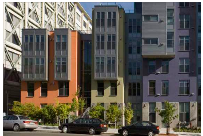
Contemporary bay windows that provide a building with unique residential-scale character and more natural light.
