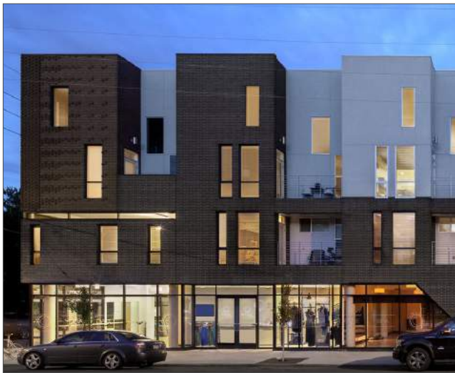
Material and color changes reinforce building massing and organization.
