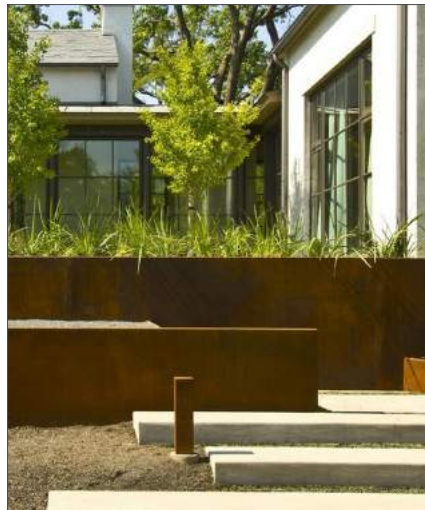
Weathering steel retaining wall at a suitable height.
