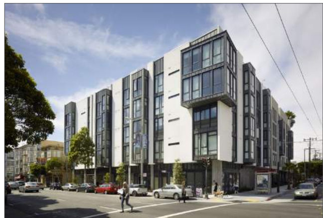
Contemporary designs often utilize pre-cast concrete and incorporate metal and glass elements.
