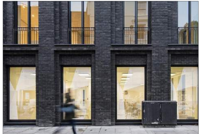
Contemporary window detailing within a simple, classic façade composition.
