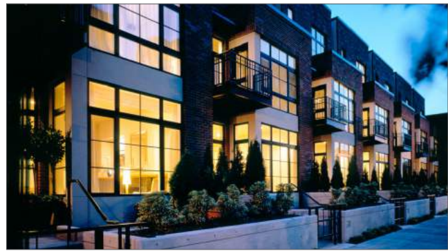
A multi-family building with two-story bay windows. The roof of the bay window is a balcony for the third floor space.
