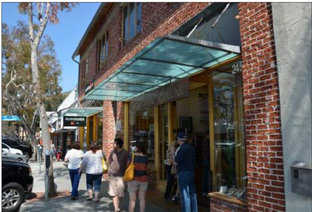
A glass awning demarcating a store entrance.
