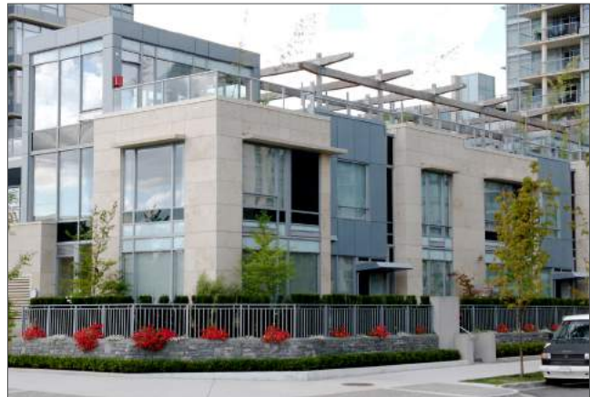
Example of a contemporary flat roof with terrace.
