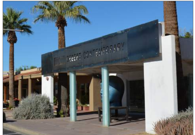
Simple, metal sign with laser-cut letters. Direct sun helps to create a legible contrast against the surface the sign is mounted on.
