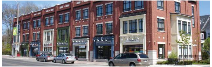
This 3-story building is clearly grouped into 25-foot bays from bottom to top, high-quality shopfronts, and careful attention to detail.
