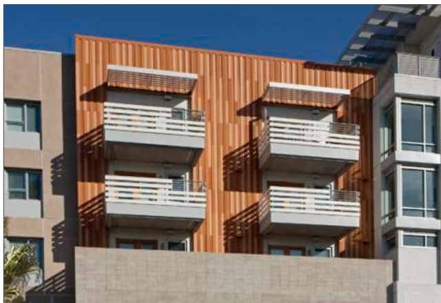
A contemporary mixed-use building with upper floor balconies and railings that shade windows and add depth.
