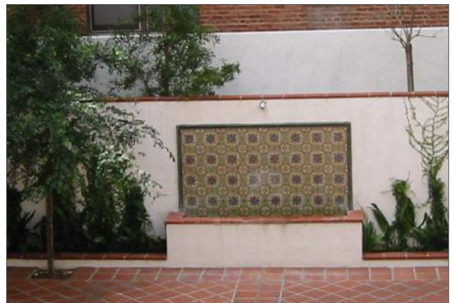
Smooth plaster walls may incorporate decorative tile or terra cotta accents. These walls also have an appropriate cap.
