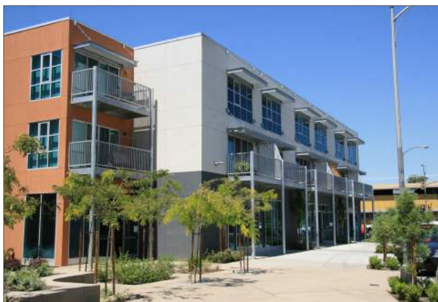
Metal awning and balconies with support poles that extend all the way down to the ground floor forming a multi-story porch.
