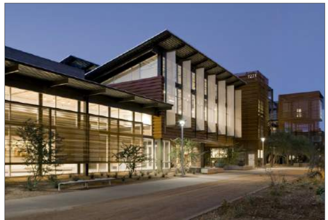
A curtain wall system paired with both vertical and horizontal shading elements.
