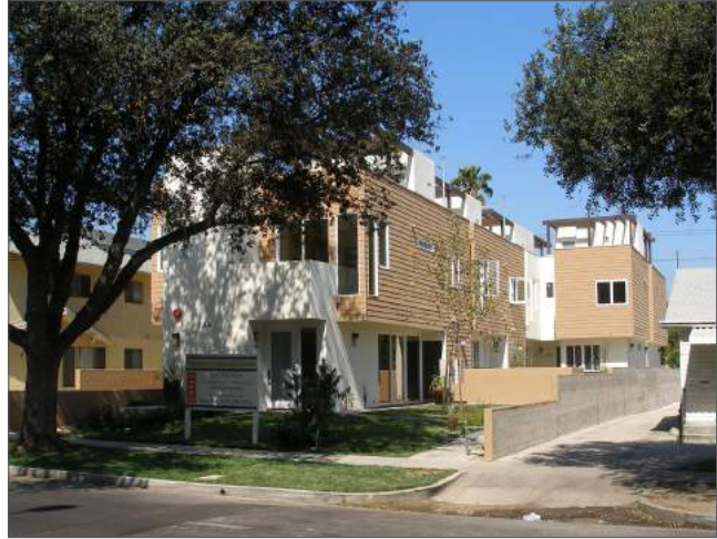
Multiple roof decks on one building.
