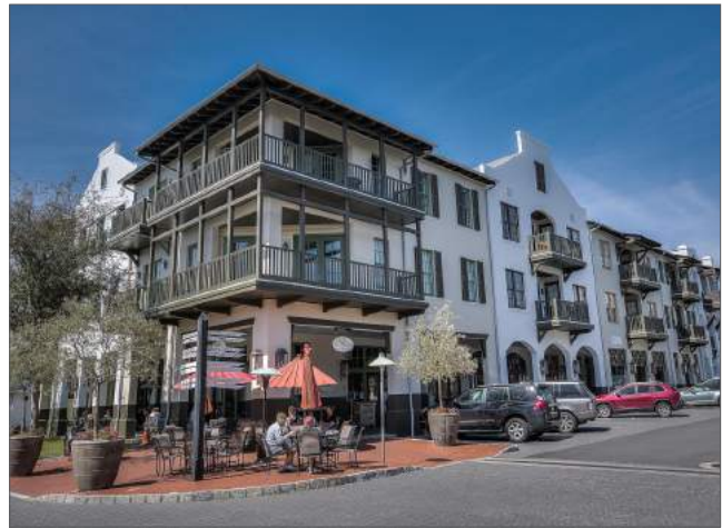
Corner balconies above a cafe.
