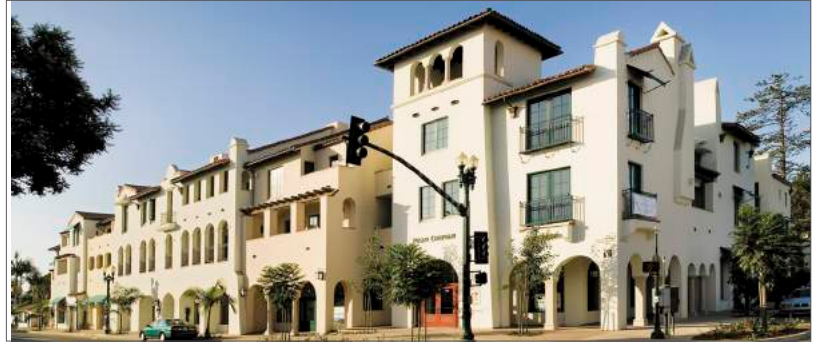
The mass of this mixed-use building is set back from the rest of the building at multiple points, with further articulation on the upper floors.
