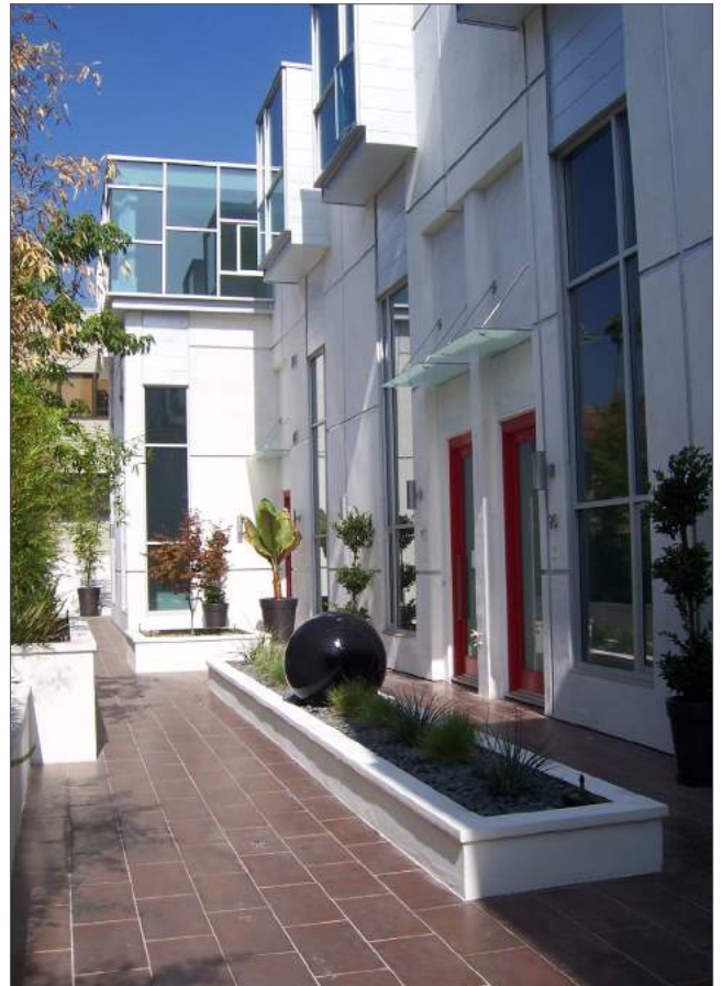
The side yard of this multi-family building provides access to adjoining units.
