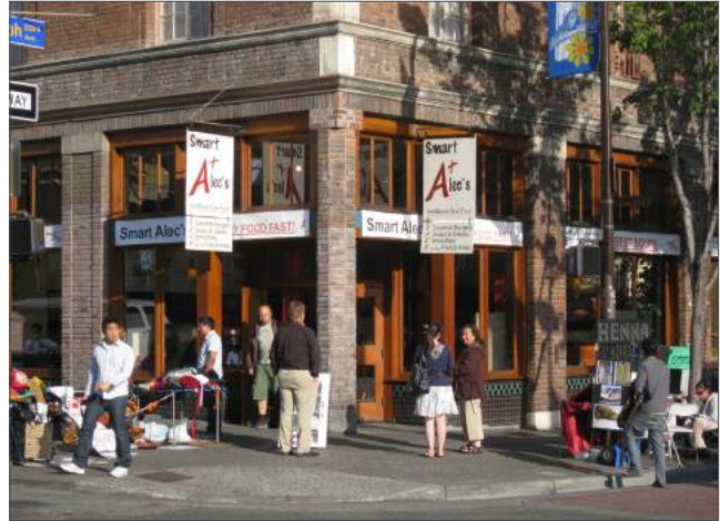
Shopfronts located at corners should create a similar character on both façades.
