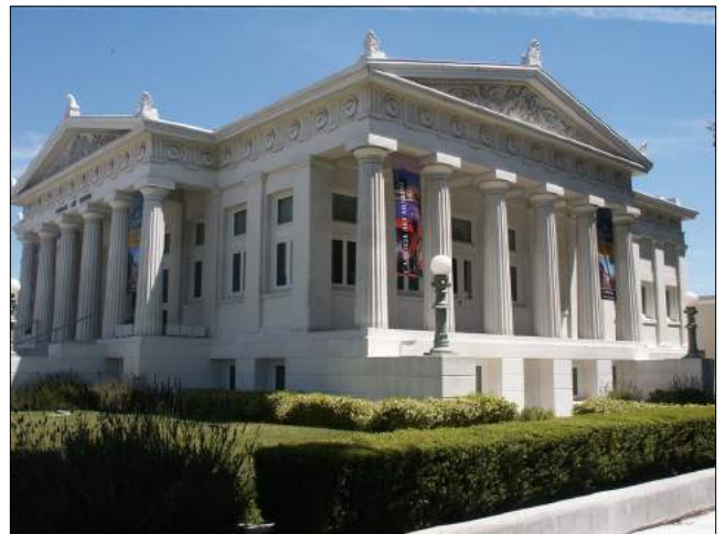
Former Carnegie Library (now Museum).
