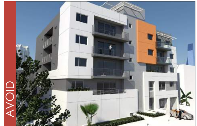
A blank ground floor frontage.
