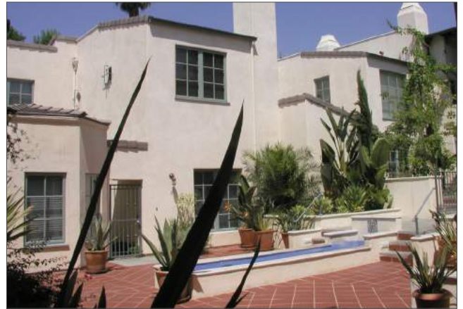
Plaster walls with pre-cast concrete caps.
