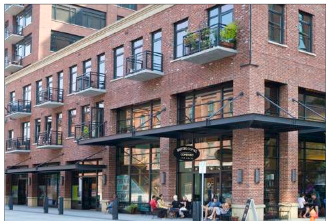
Concrete and masonry building with simple openings and industrial metal awnings, canopies and balconies give this building an attractive, elegant character.
