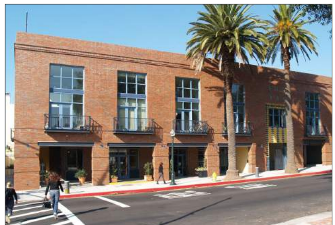
A brick building with an articulated parapet and wrought-iron balconies.
