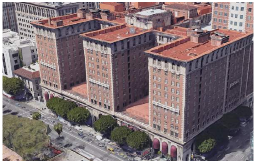
The Millennium Biltmore Hotel in Los Angeles is an E-shaped building that uses Courts above the base to provide light and ventilation to its rooms, as well as effectively break up the massing along the street.
