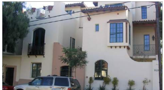
Architectural recessions help modulate the scale (vertical and horizontal) of these attached rowhouses to house-form.
