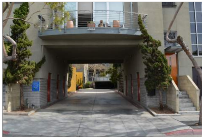
A car entry into a parking court can be subtly integrated with existing residential elements such as balconies.
