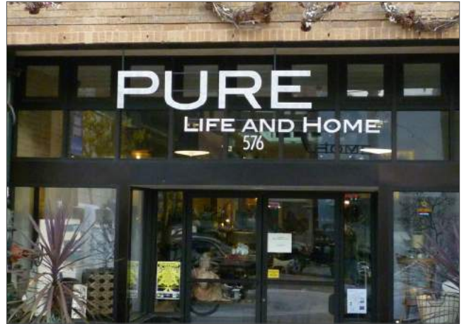
Wall signs may be located within the transom area of the shopfront.
