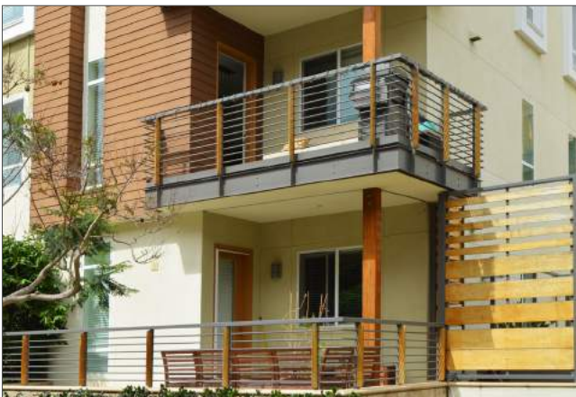
A wood balcony supported by extended beams.
