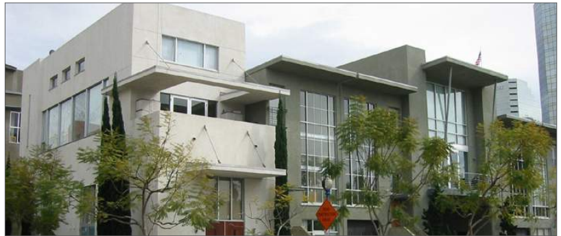
A multi-family building where the massing is vertically broken down into smaller volumes.
