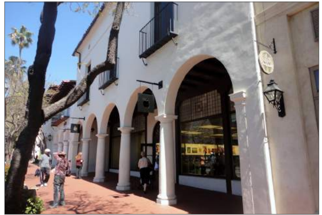
Large areas of glazing should be recessed and shaded as opposed to tinted.
