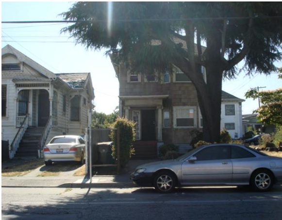
3608 West Street, Oakland
