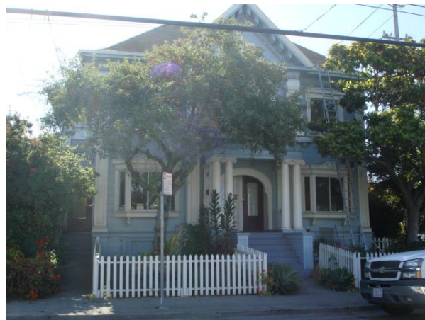
4504 West Street, Oakland
