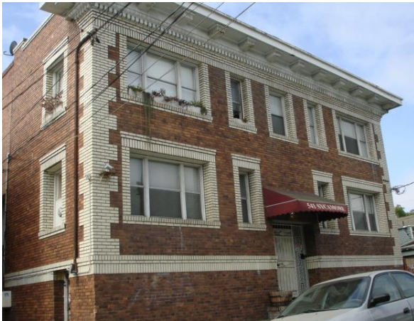
541 Sycamore Street, Oakland
