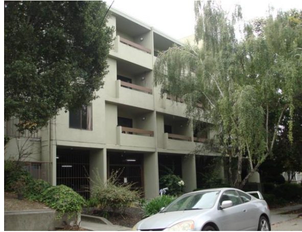
424 Orange Street, Oakland
