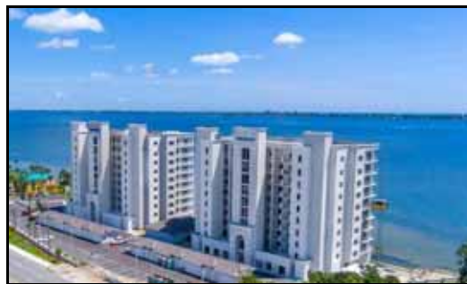
Paramount Condominium Project
