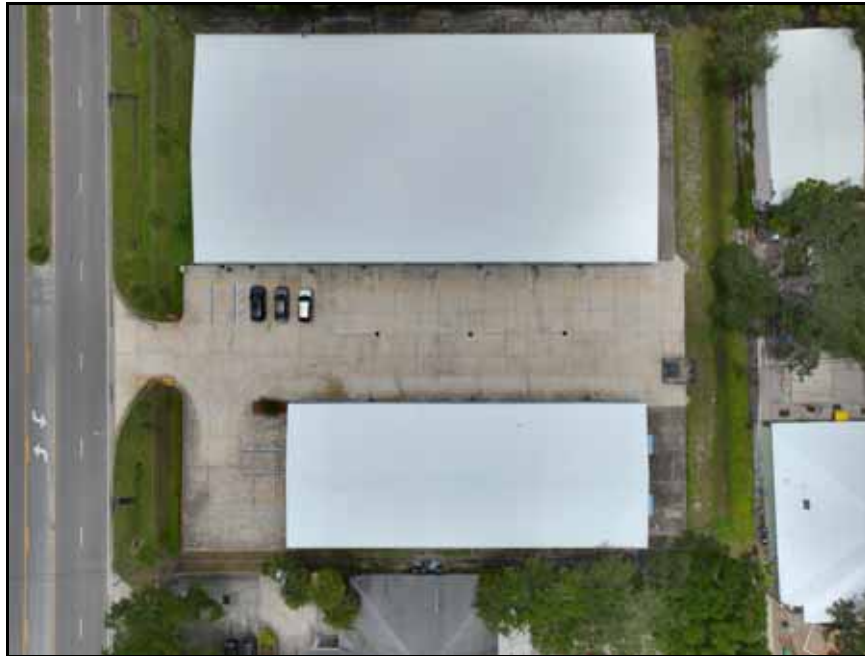
Aerial (Eagle View) Photograph of Subject Roofs After Replacement in 2024 & 2025
