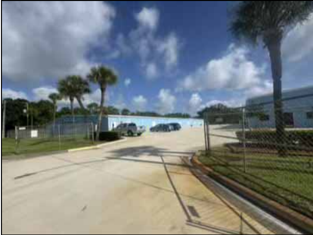
Subject Front (Ingress/Egress) – South Elevation
