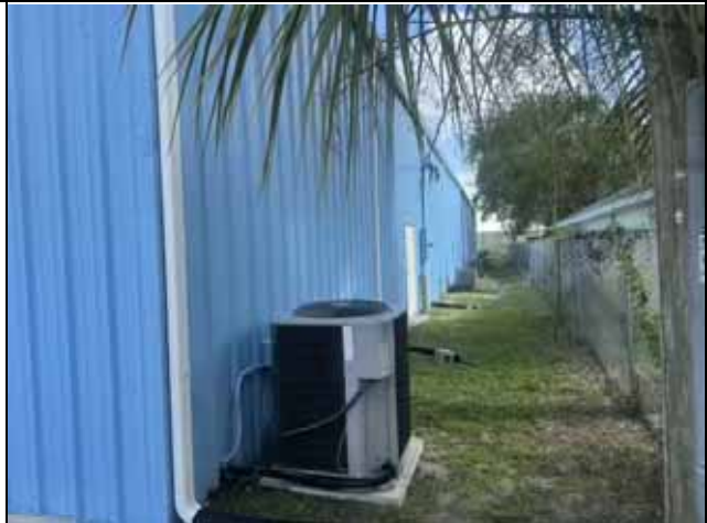
Side – 1350 Lake Washington Rd. (Southeast Corner)
