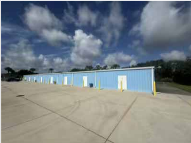
Side – 1360 Lake Washington Rd. (Northeast Corner)
