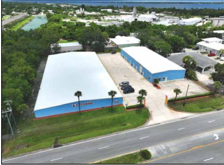
Eagle View of A1 Storage (1350 & 1360 Lake Washington Rd.) Facing Northeast
