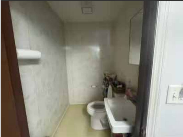
Office Bathroom – 1360 Lake Washington Rd.
