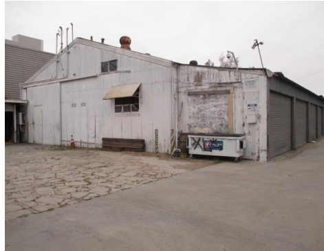
Metal Building - East Elevation.
