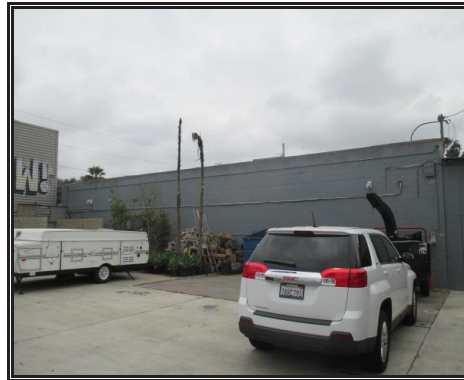
Concrete Block Building - north elevation.
