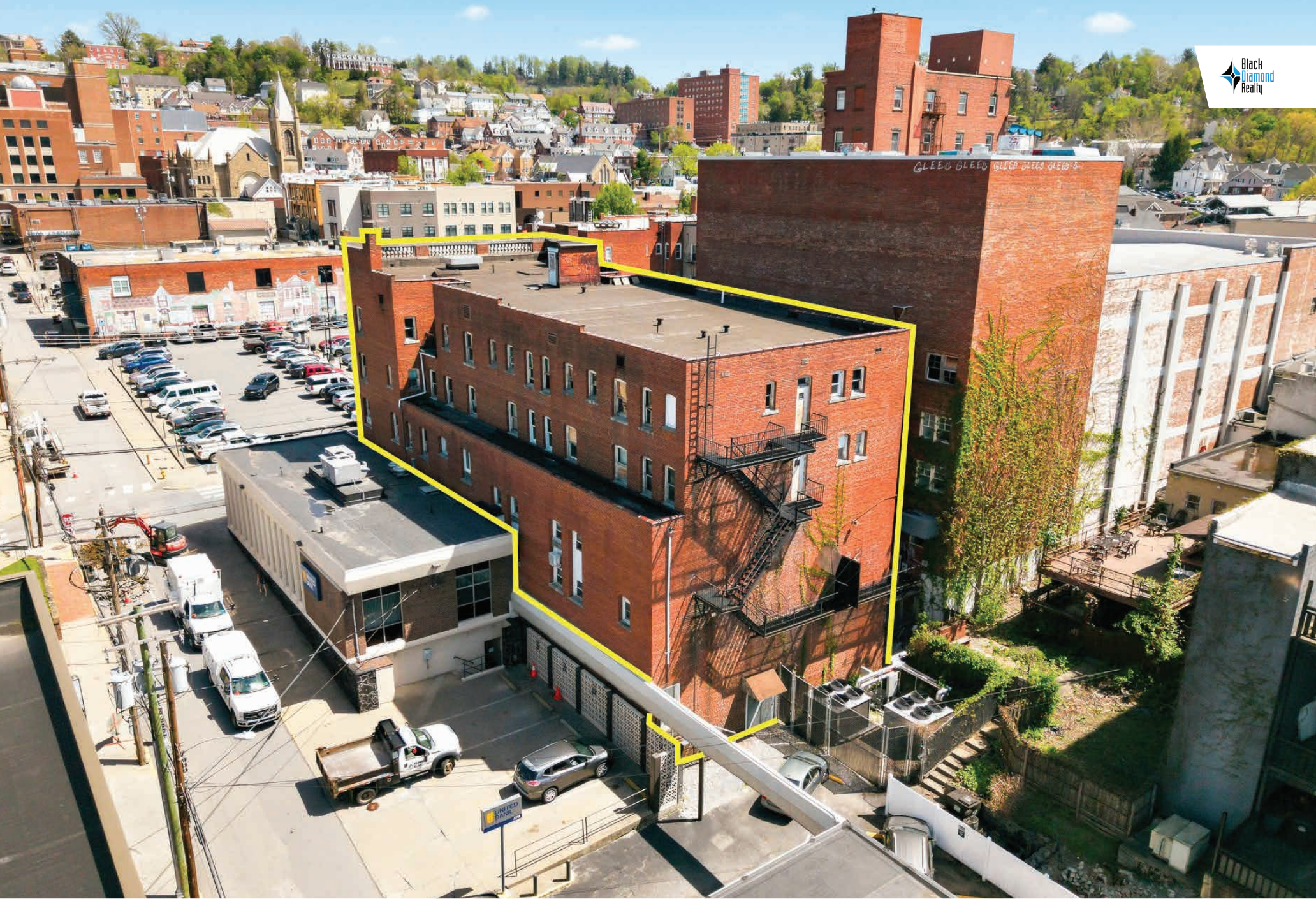
Exterior Back of the Building.
