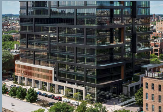
Fulton Labs at 400 N. Aberdeen, Chicago Trammell Crow Company 425,000 SF – Delivered 2022
