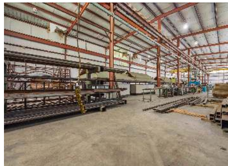
Building B steel shop
