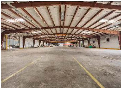
Building A warehouse
