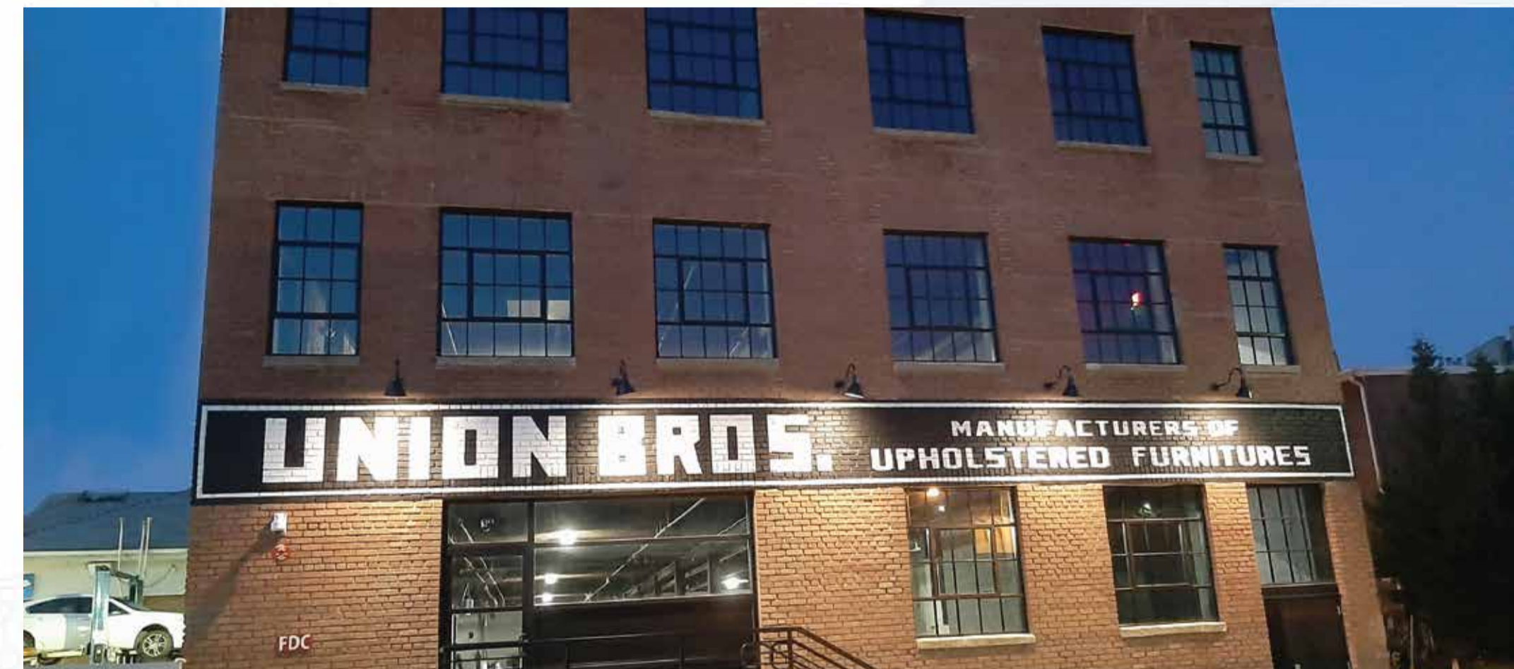
UNION BROS. BUILDING POST RENOVATION
