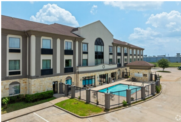
Main building elevation with pool overview
