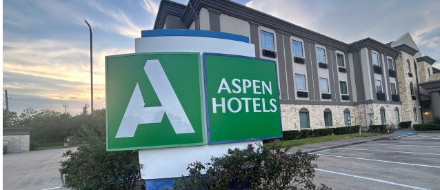
Exterior frontage and building identity
