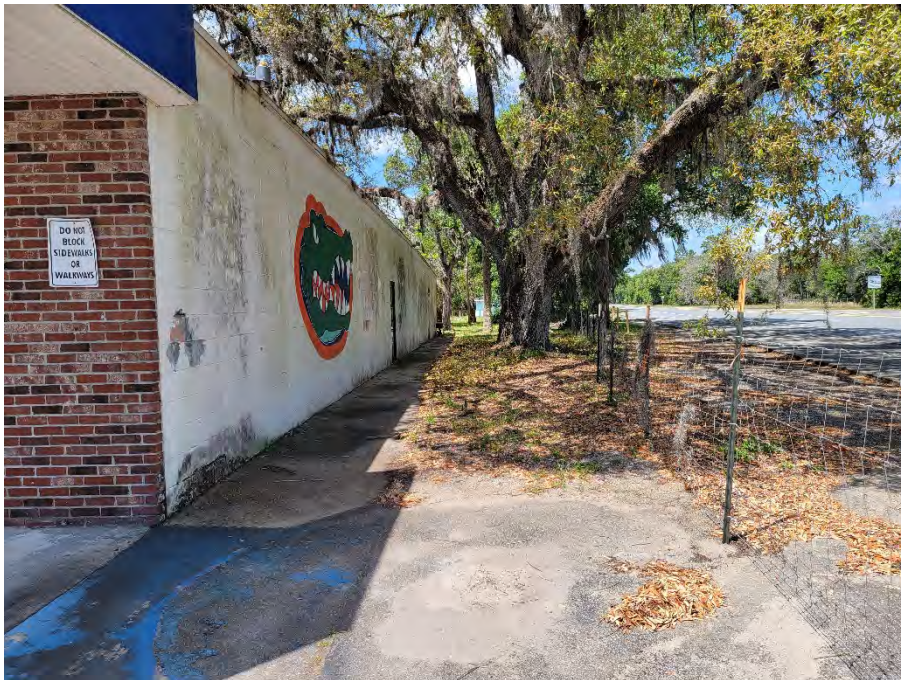
Photograph 7. Subject property building, northern façade.
