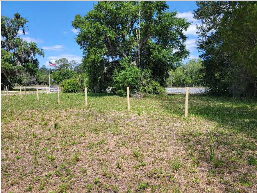
Photograph 11. One of three septic tank drainfields on the subject property, surrounded by bollards to prevent access.
