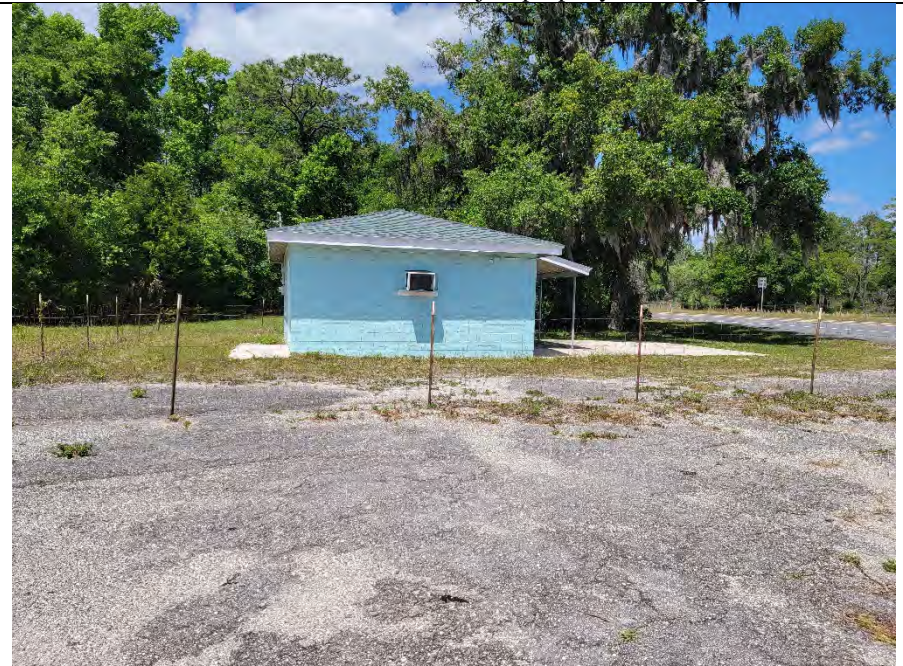
Photograph 12: North adjoining Clay County Sheriff's Office substation, 6026 Kingsley Lake Drive.
