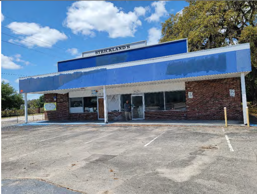
Photograph 1. Subject property building.
