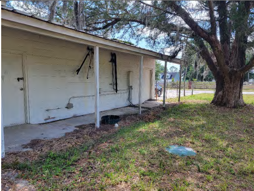
Photograph 9: Western building façade.
