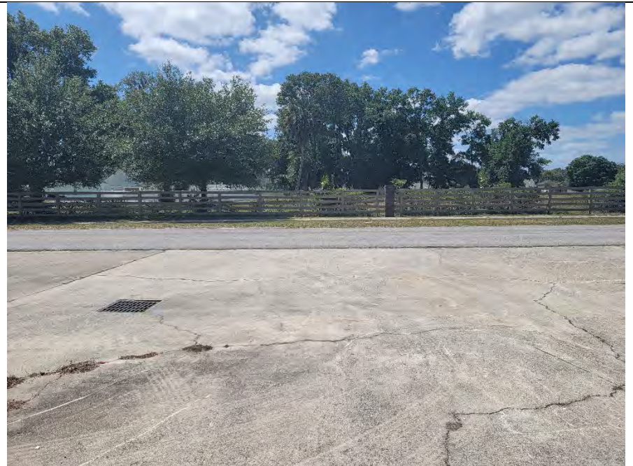
Photograph 20: South adjoining property.
