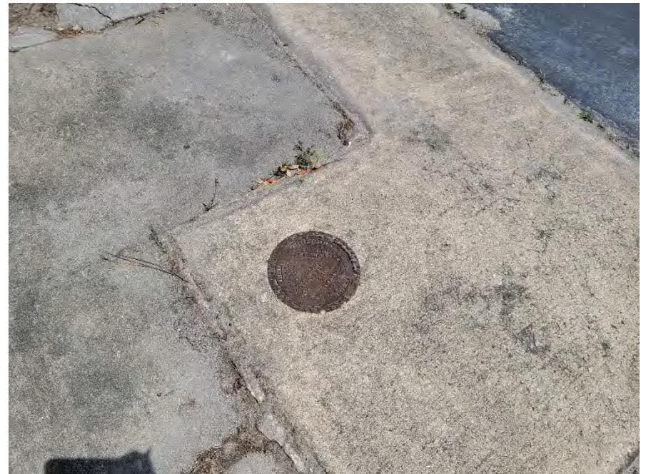
Photograph 4. Typical monitoring well on the vicinity of the fuel tanks and pumps.
