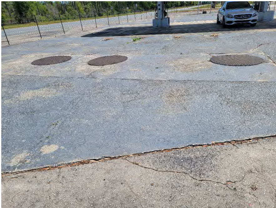
Photograph 3. Fuel tanks on the east side of the subject property building.
