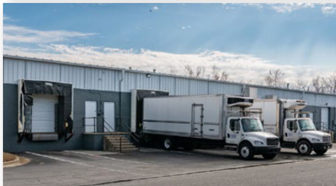
205 Creek Ridge Rd | Loading Areas
