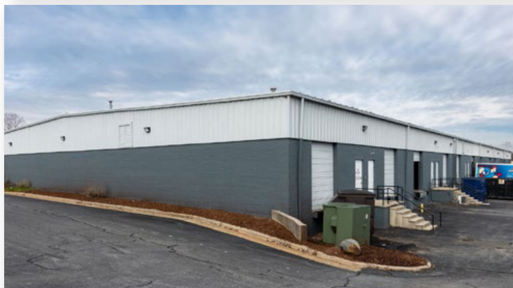
103 Creek Ridge Rd | Loading Areas
