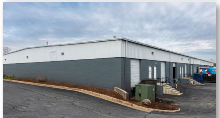
103 Creek Ridge Rd | Loading Areas
