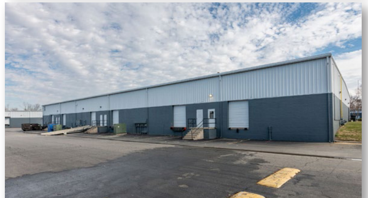
209 Creek Ridge Rd | Loading Areas
