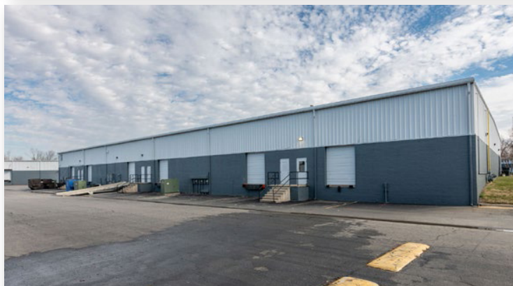
209 Creek Ridge Rd | Loading Areas
